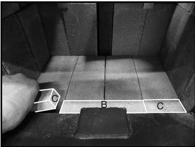
Figure 31: Narrow front bricks in place.
