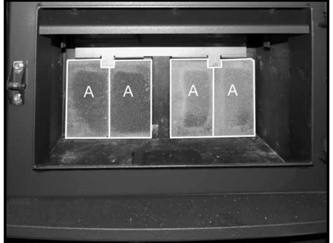
Figure 26: Remaining rear wall firebricks in place.
